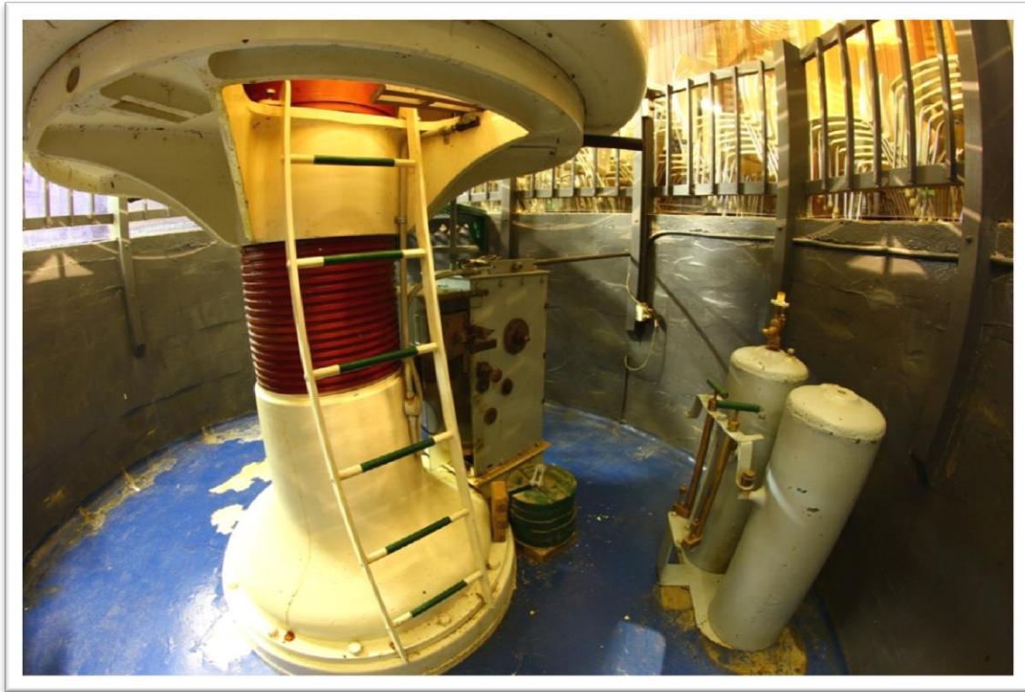
Figure 2 South Solitary Lighthouse pedestal, pressurised water and kerosene tanks, clockwork and weights. The ladder leads up to the inside of the optic. The optic needed to be accommodated in a pit due to its height, Coffs Harbour Regional Museum. Photo: Dave Senior
