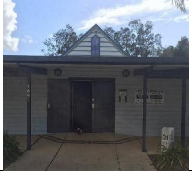
Figure 30. Entrance door through which SSILO will need to be removed in parts
