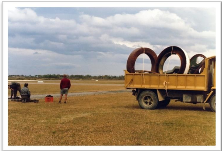
Figure 4: South Solitary Lighthouse pedestal being loaded onto a truck at Coffs Harbour Airport, September 7 1977. Photo courtesy of Lyndon O'Grady
