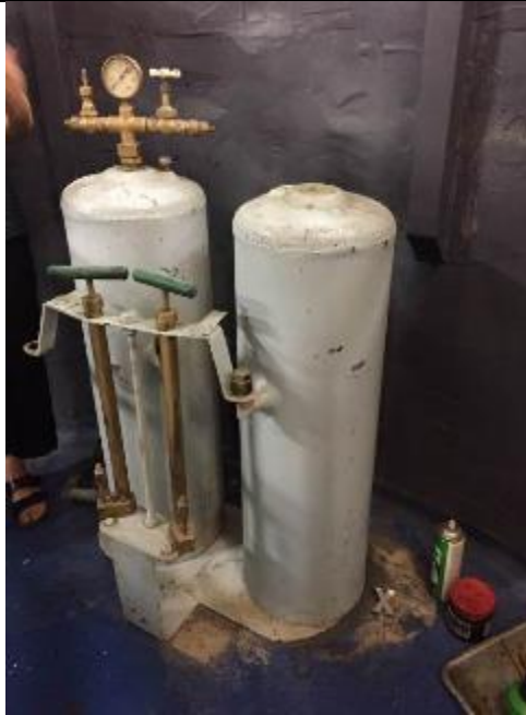
Figure 44. Kerosene and water cylinders
