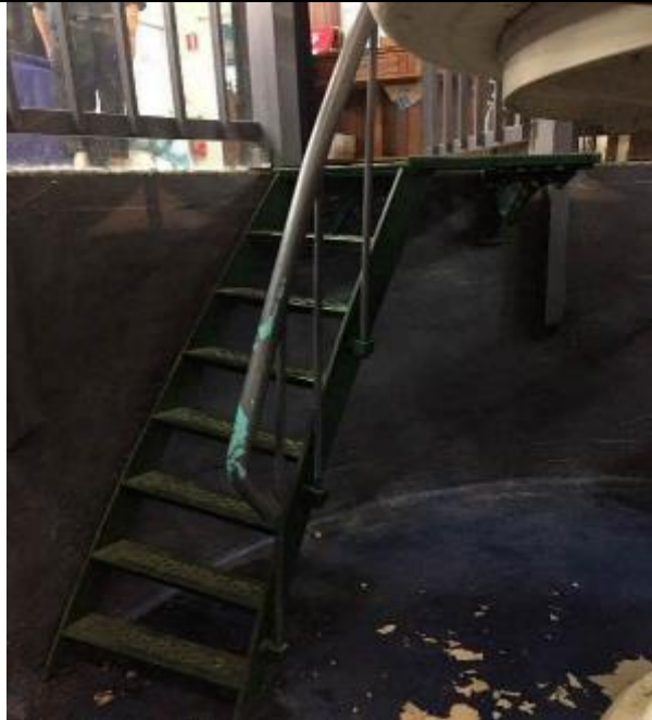
Figure 35. Entrance stairway to pit
