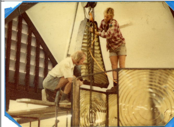
Figure 19. Reassembling the lighthouse optic in the new museum
