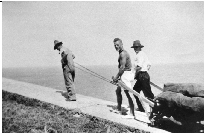
Figure 11. South Solitary Island Light Provision Day 1931. L-R Alf Smith, Wilfred Tulk, Phil Padden, Coal bunkers in the renowned 3 man-power truck
