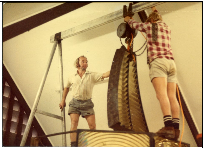
Figure 18. Reassembling the lighthouse optic in the new museum
