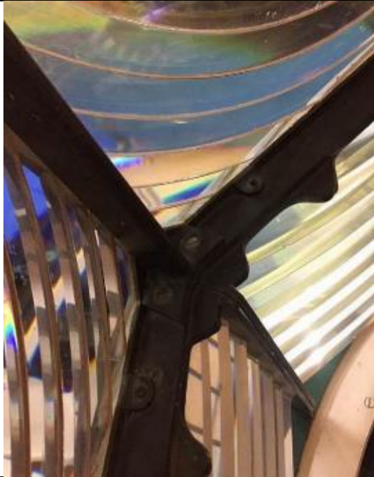
Figure 40. Internal screw fixings
